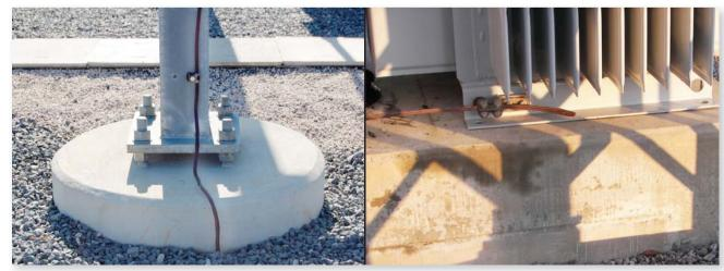
Thieves will steal coils of copper wire if they can get them; otherwise, they will go after the copper making up the grounds (left). Often, the criminals will just cut the sections off (right). The more enterprising thieves will tie the ground to a truck and see how much can be exposed before cutting.
